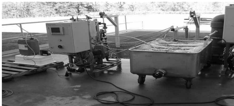
Figure 1. Microfiltration modules submerged in tank and necessary pumps and cleaners in place at plant.
